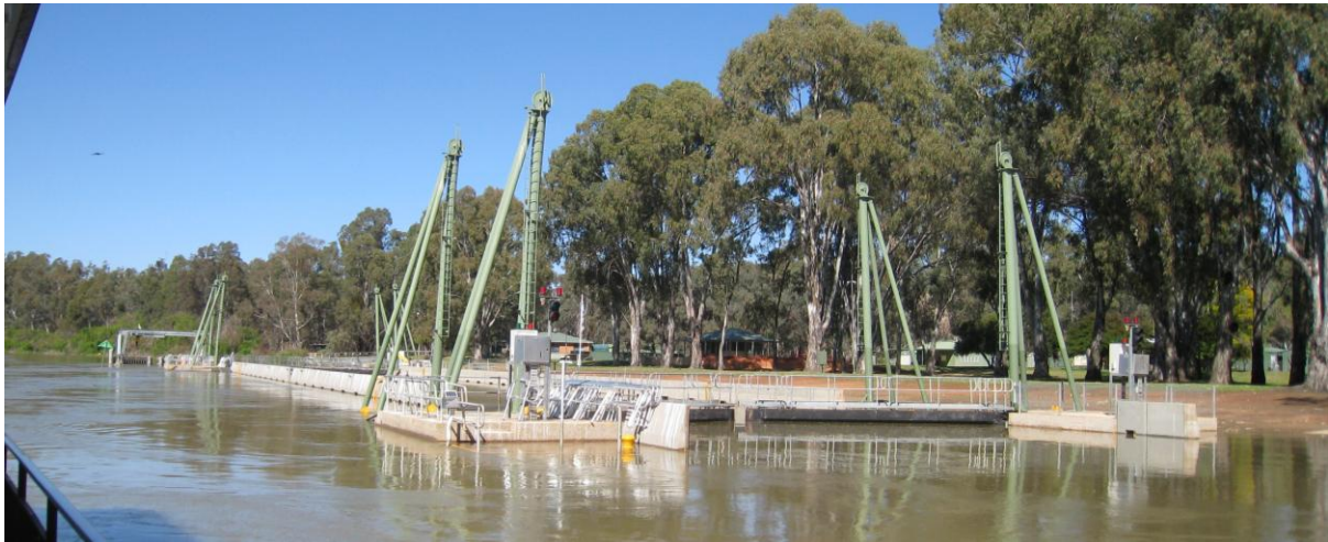
Flooded Lock 7 with open Navigational Pass to left
